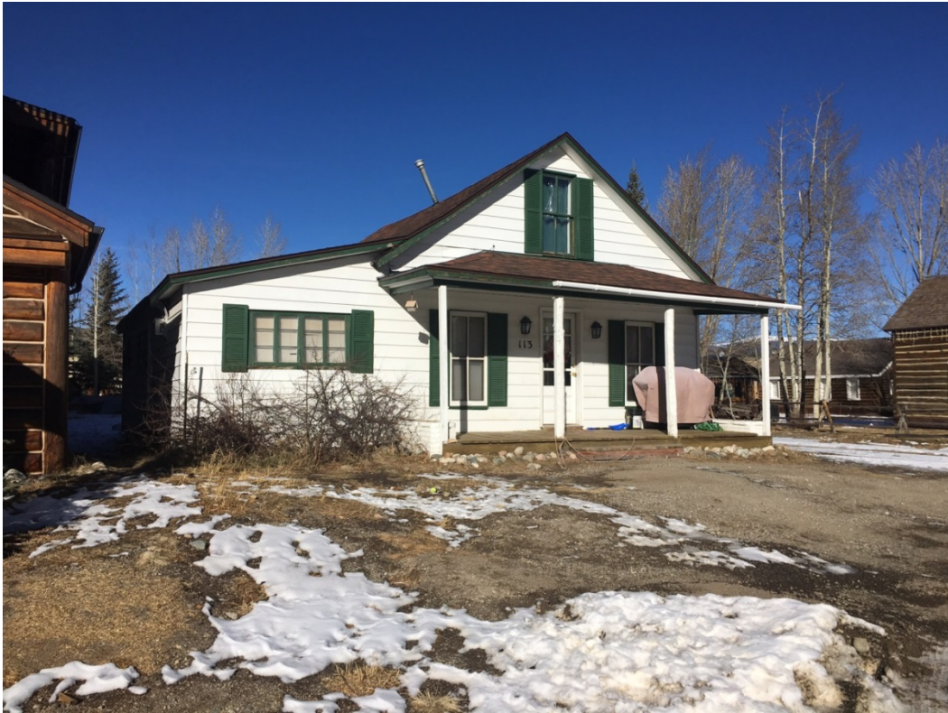
View looking north 12.12.17
