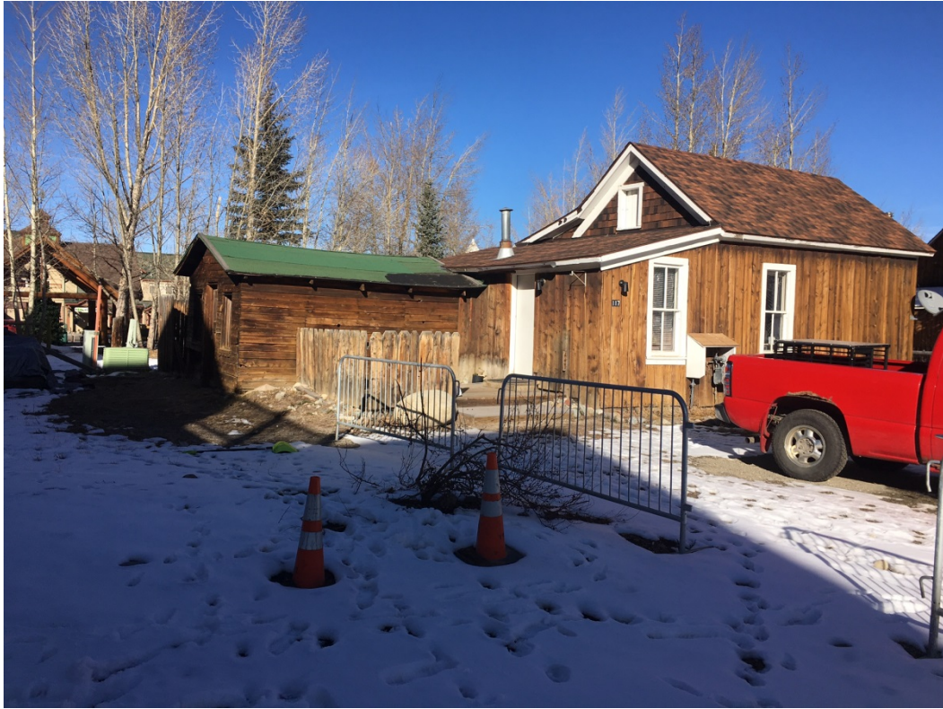
View looking northeast at 117 Granite Street Dec 12.12.17
