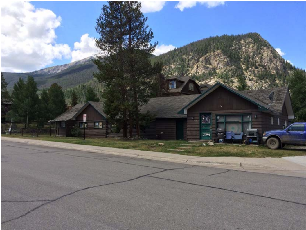
East elevation viewed from South 4 th Avenue (8/13/15)
