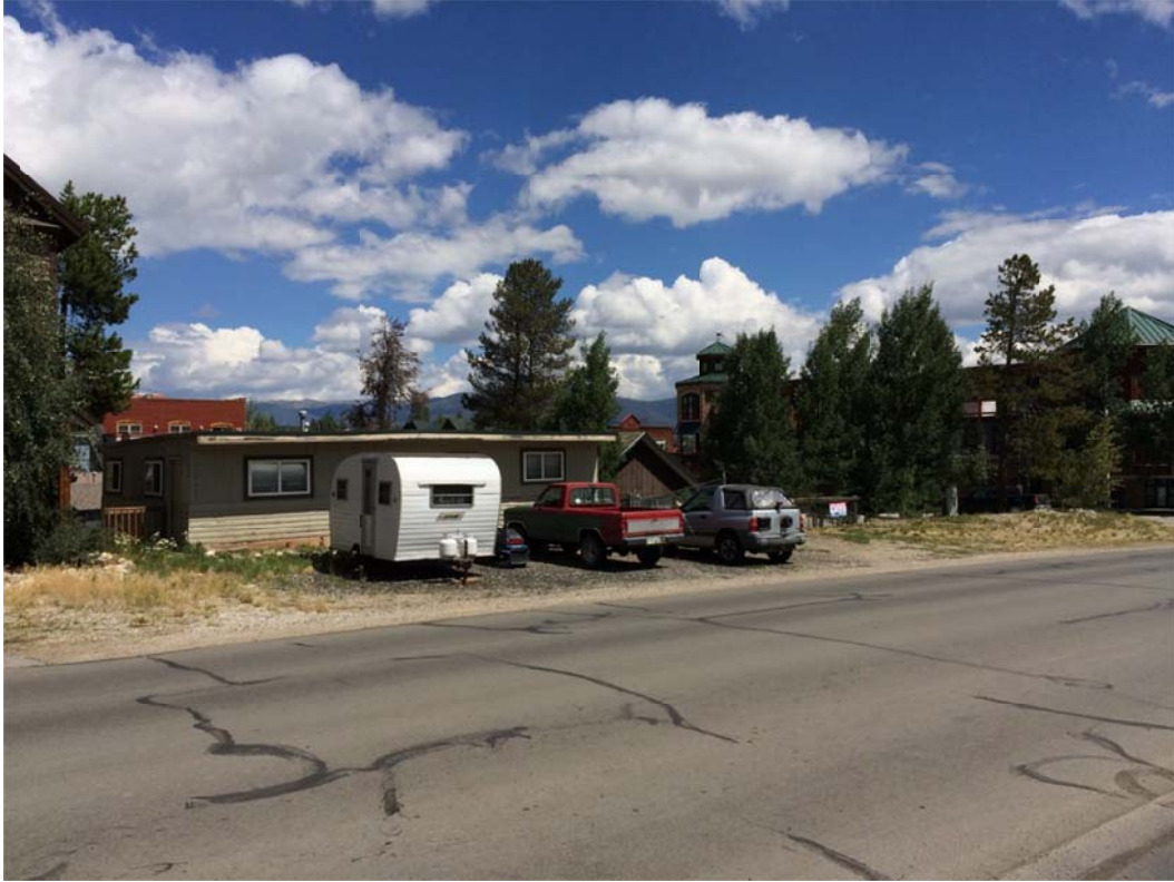
Southwest elevation viewed from Granite Street (8/13/15)
