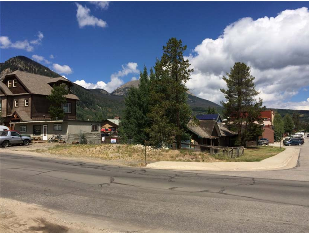
Southeast elevation viewed from Granite Street (8/13/15)
