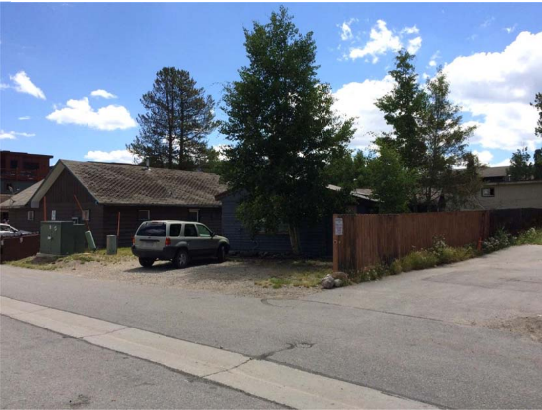
Northwest elevation viewed from Granite Street Alley (8/13/15)
