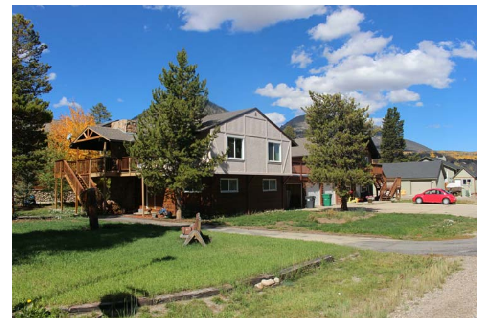
EXISTING RESIDENCE AND DUPLEX, VIEW FROM SOUTH-EAST
