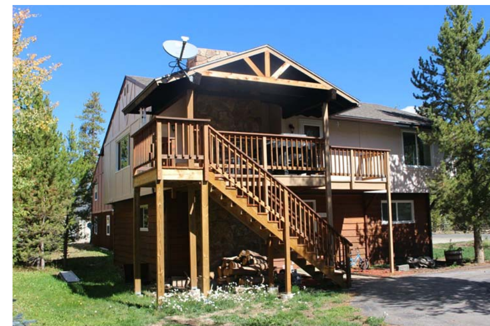
EXISTING RESIDENCE, VIEW FROM SOUTH
