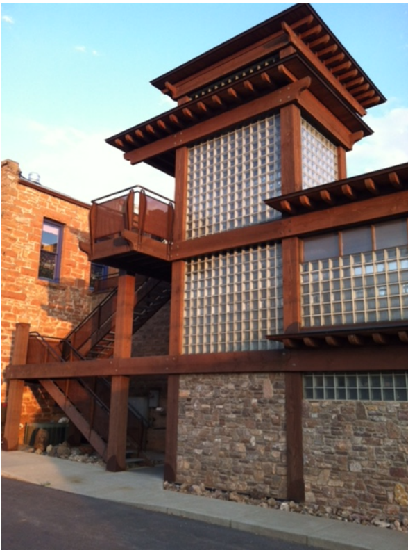
Heavy Timber Posts/Beams and Soffits:
