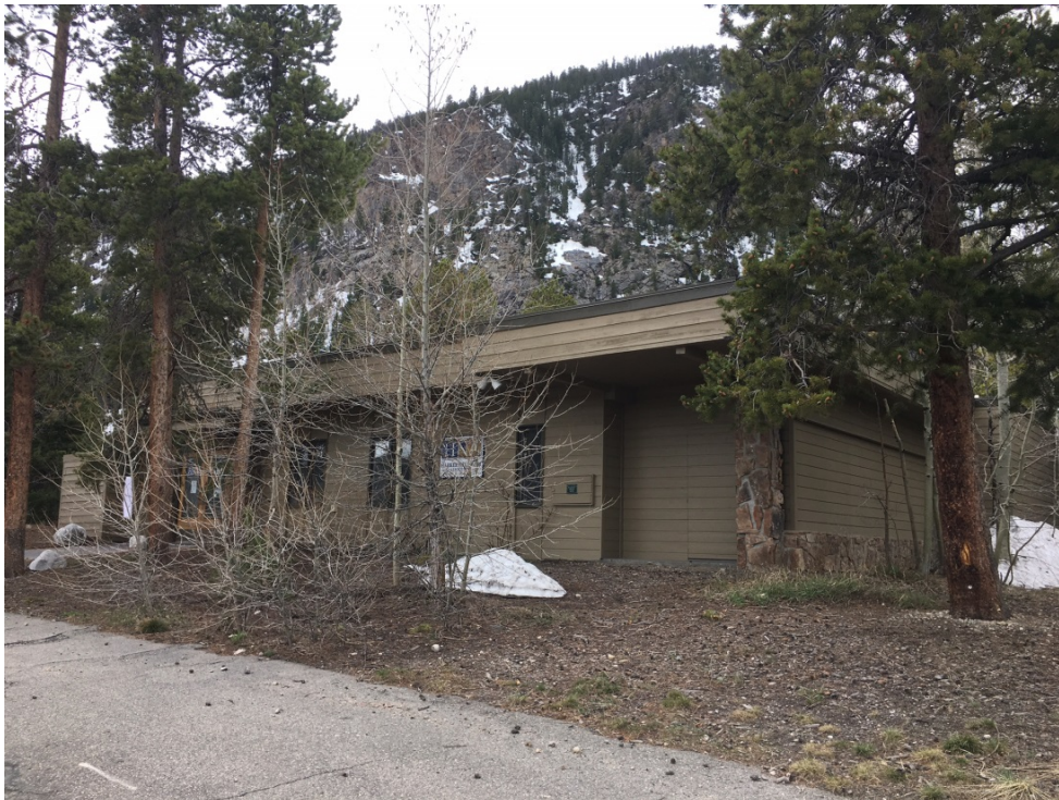
View from northeast corner (April 20, 2017)
