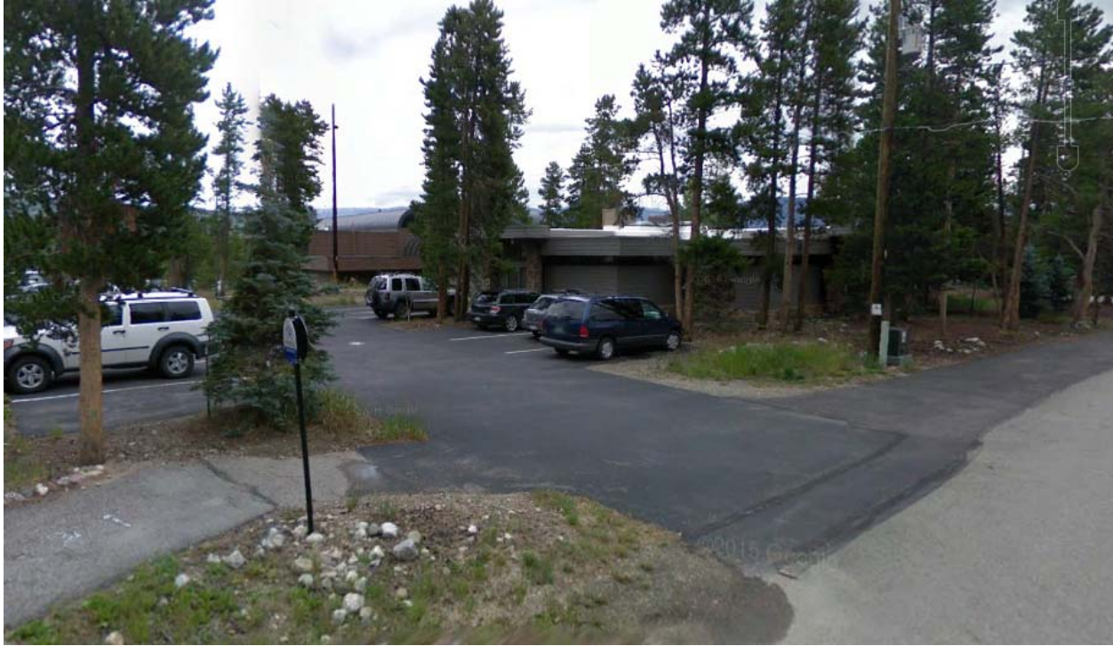
View from southwest corner (Google Earth, August 2008)
