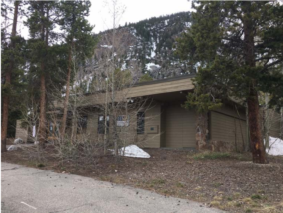
View from northeast corner (April 20, 2017)
