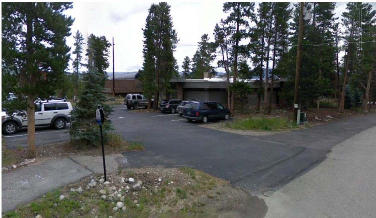
View from southwest corner (Google Earth, August 2008)
