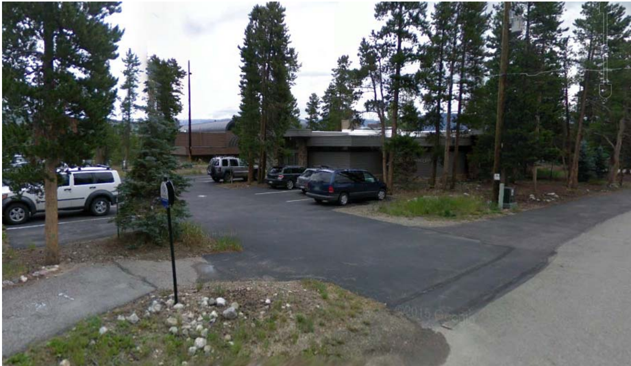
View from southwest corner (Google Earth, August 2008)
