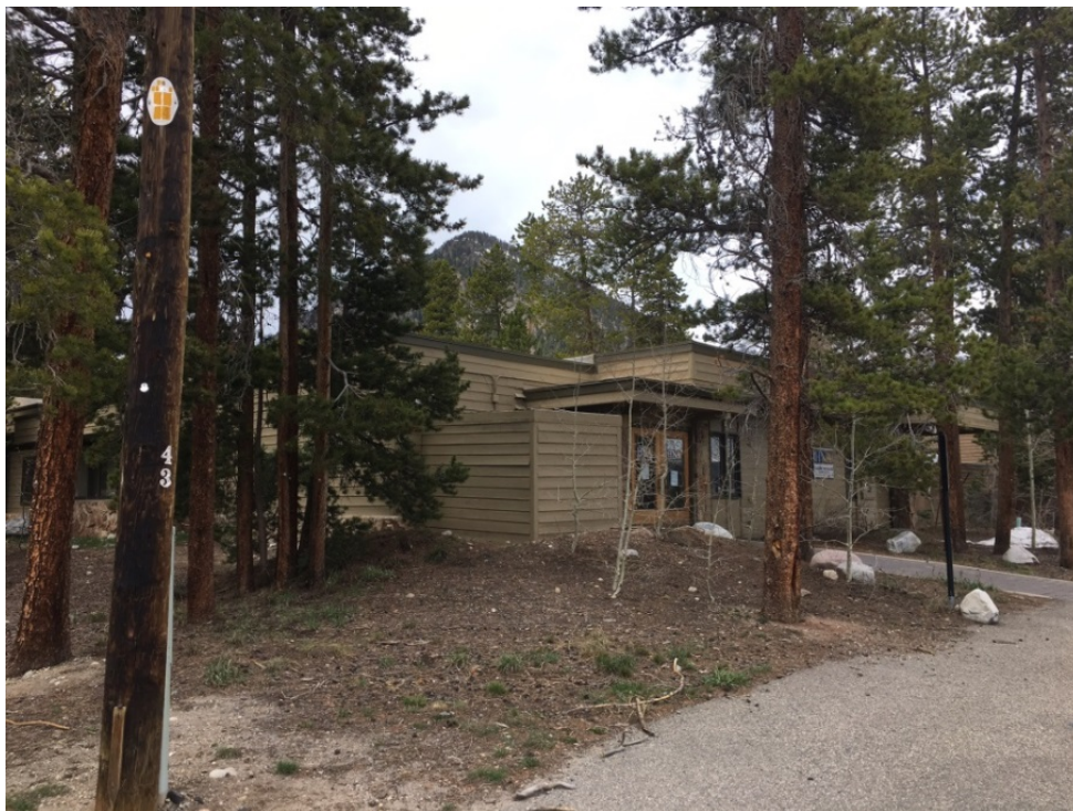
View from southeast corner (04/20/2017)
