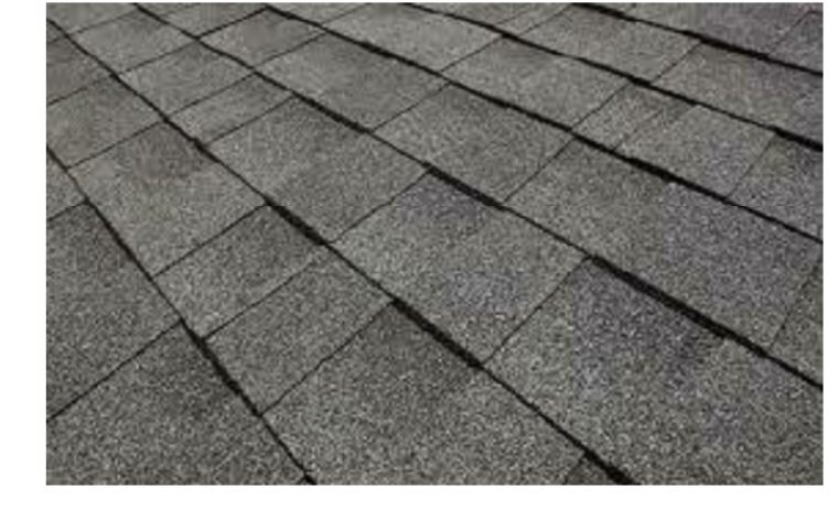
ASPHALT SHINGLE ROOFING WEATHERED WOOD
