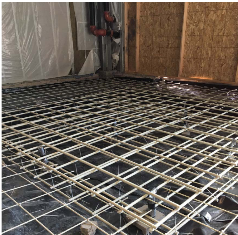
Steadman Clinic at 226 Lusher Court (fiberglass rather than metal rebar for concrete reinforcement under an MRI machine)
