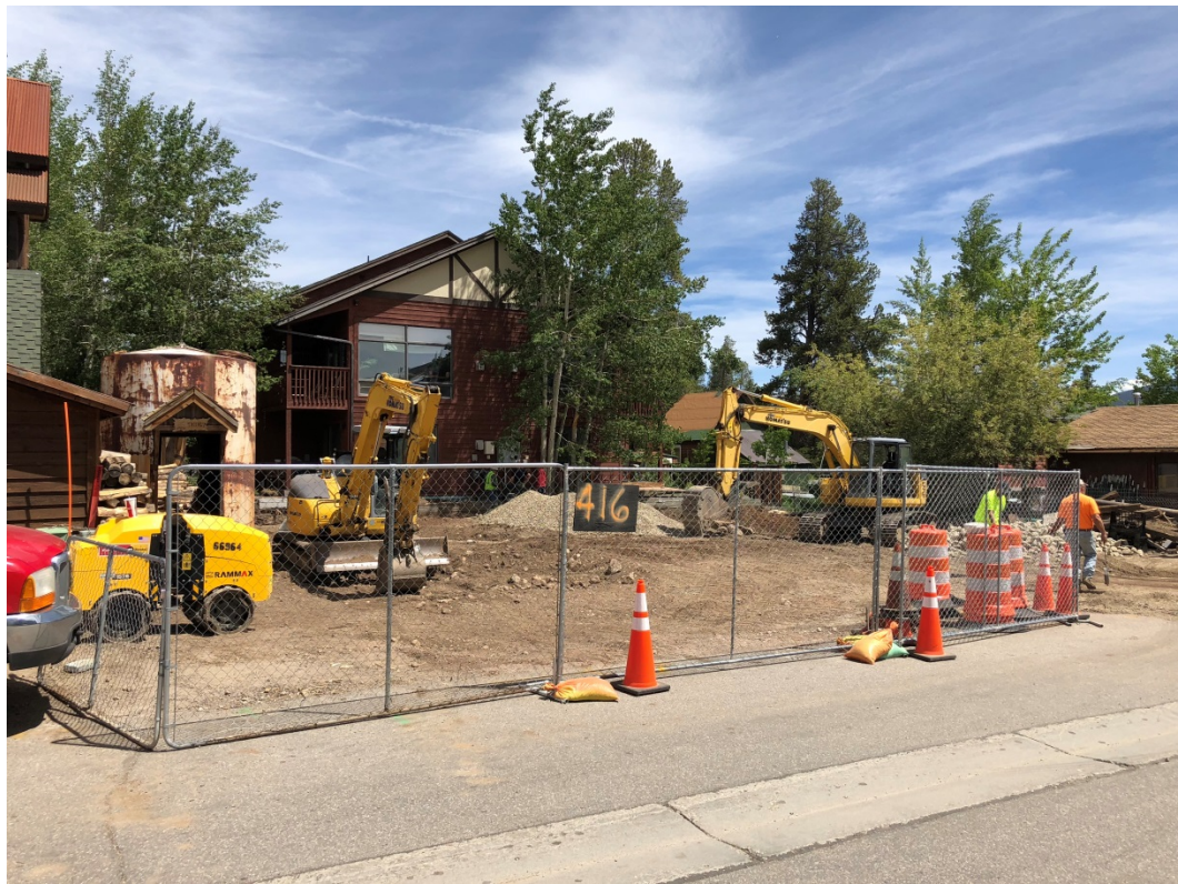
Alley Shacks Duplex at 416 Galena Street Alley
