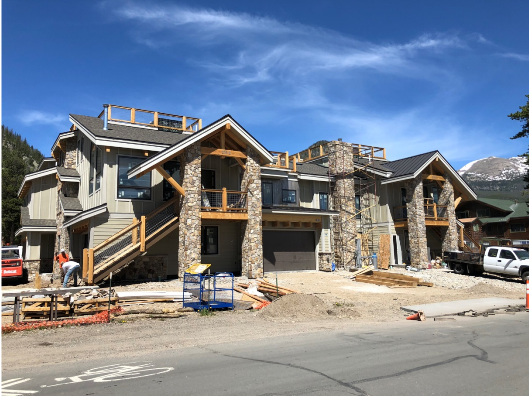
Mae Belle Creek Townhomes at 215 South 2 nd Avenue – closing in on the finish line.
