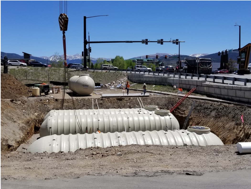
Kum & Go at 55 Lusher Court 3 – 12,000 gallon tanks and 1 – 20,000 gallon tank installed.
