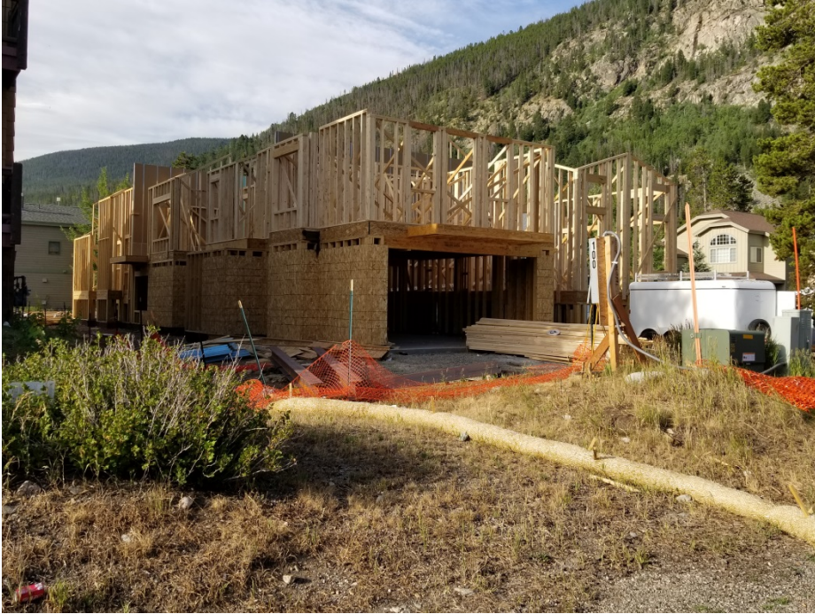
Mattox Townhomes at Granite and Madison going 2 nd floor verticle. This project has done a good job at managing their construction site to minimize impact to the right of way and neighbors, dust, and storm water control.
