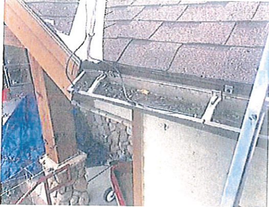
Loose gutter
