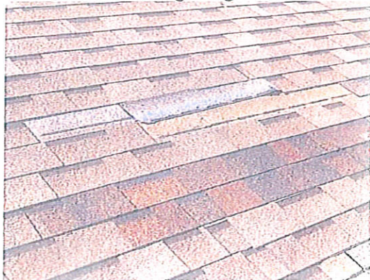
Missing shingles
