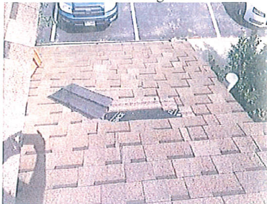
Missing shingles
