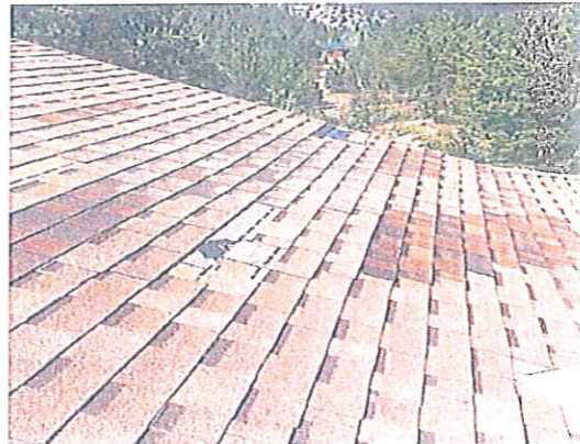
Missing shingles
