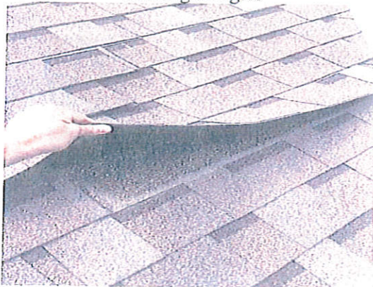
Missing shingles
