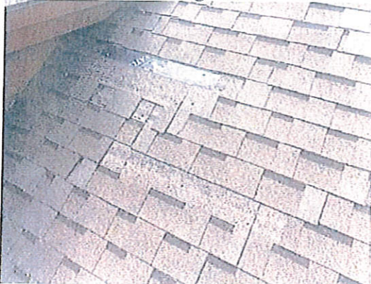
Missing shingles
