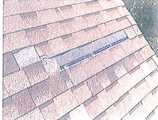
Missing shingles
