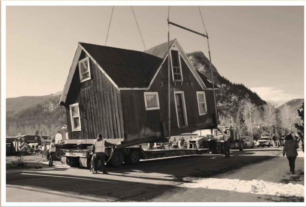
Excelsior Mine Office Building Preservation Project 2018
