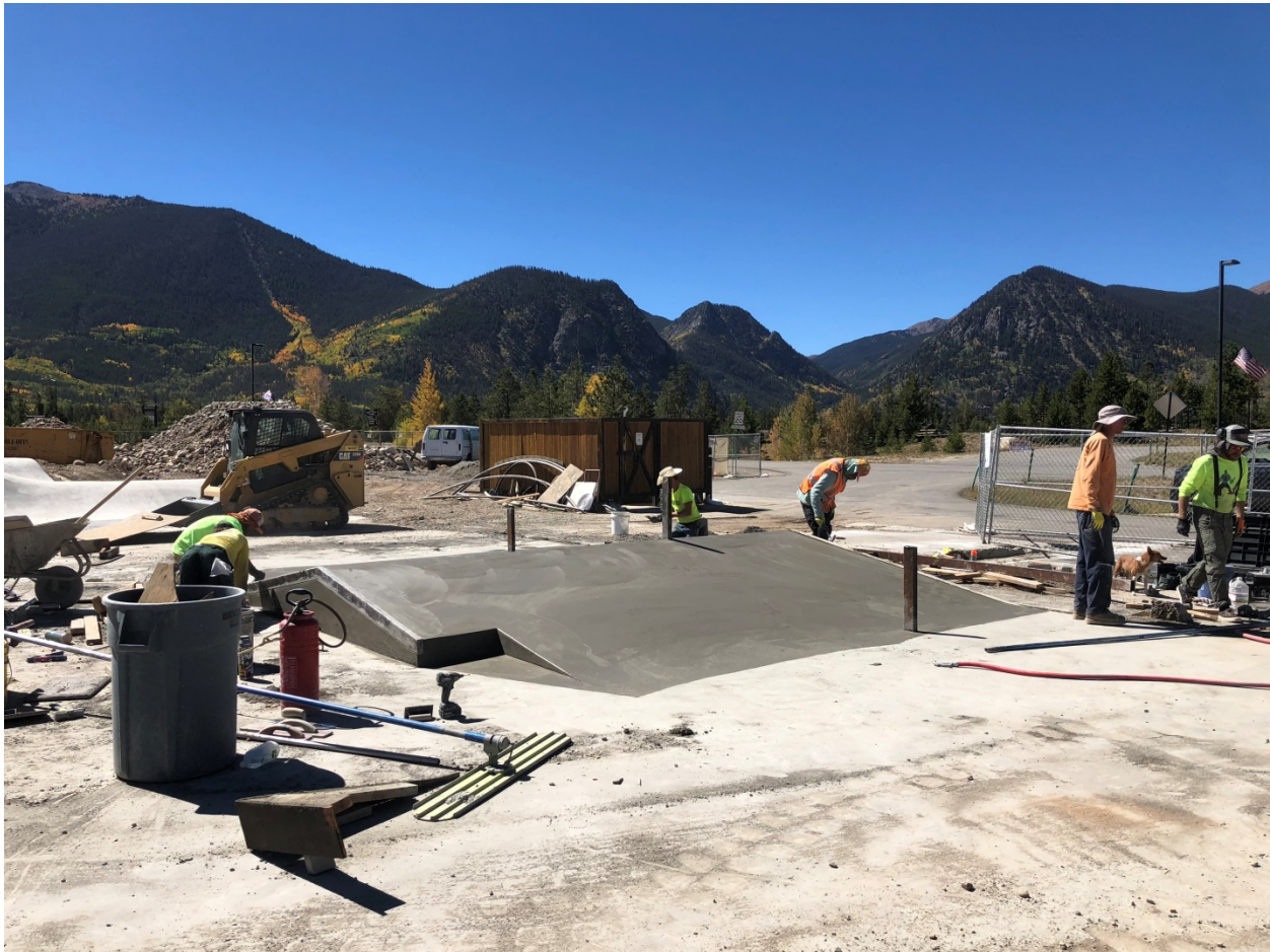
Photo 1: Skate Park – Street Course Concrete Pour on 9/13/18.
