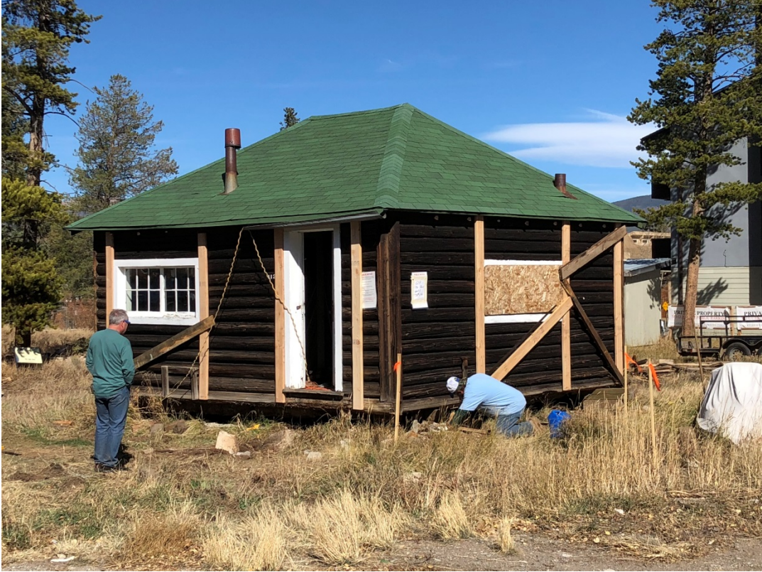
Deming Crossing Project at 112 North 5 th Avenue
