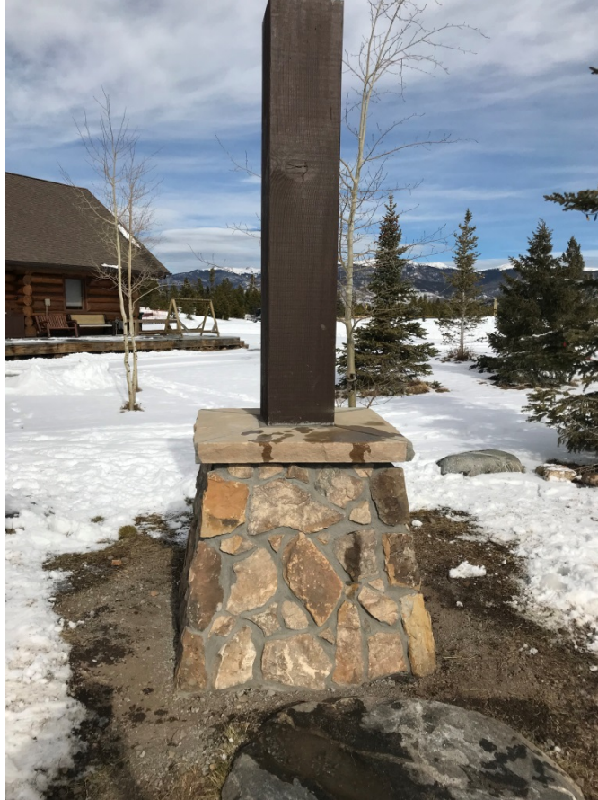
Photo 5: New Wayfinding Sign Base
