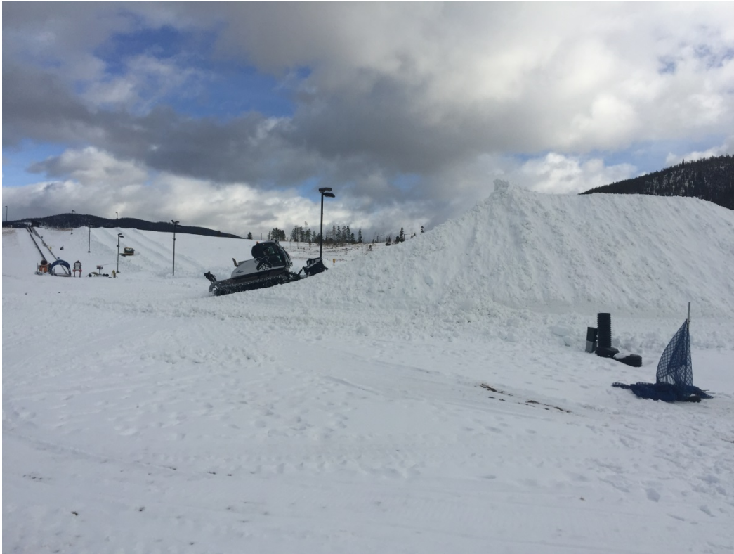
Photo 2: Tubing Hill Construction – 11/21/17
