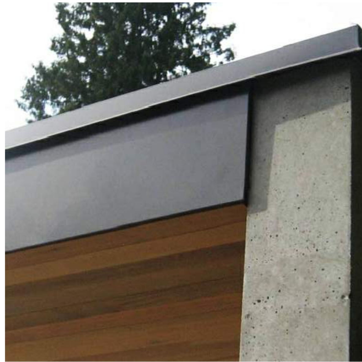
DARK BRAKE METAL TRIM - FASCIA, GUTTERS, DOWNSPOUTS, ETC (BARRIDGE OR SIM)
