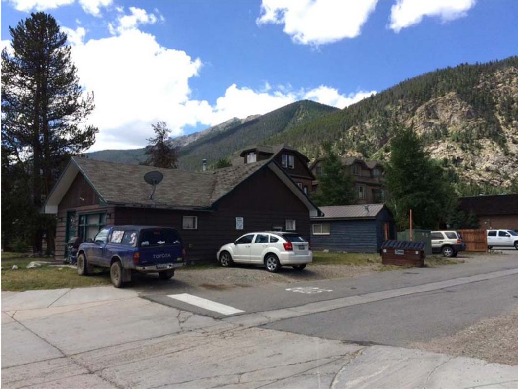
Northeast elevation viewed from South 4 th Avenue (8/13/15)
