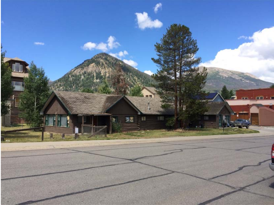
Southeast elevation viewed from South 4 th Avenue (8/13/15)
