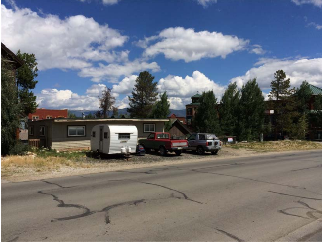
Southwest elevation viewed from Granite Street (8/13/15)
