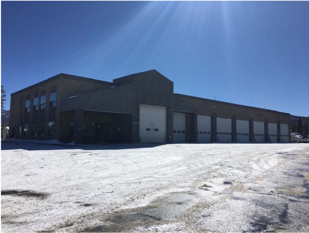
Northwest Corner of Existing Structure
