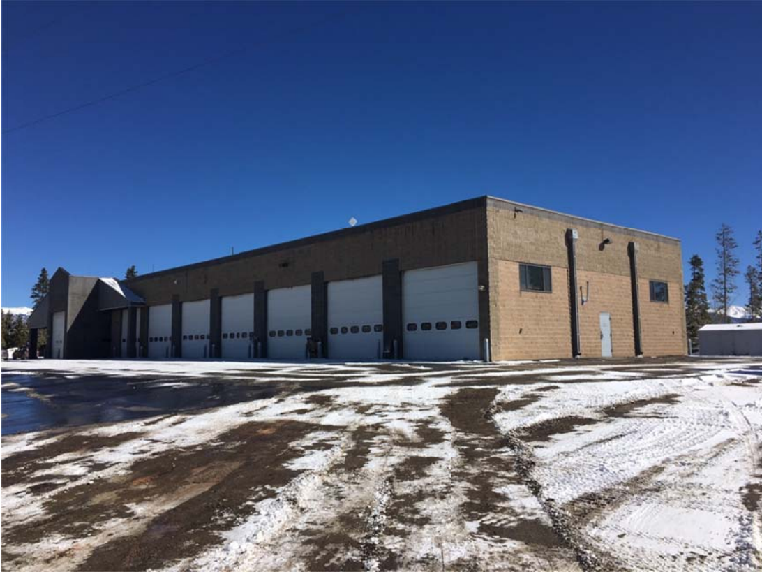
Southwest Corner of Existing Structure
