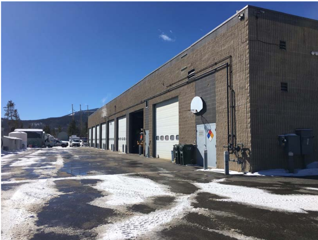
East Façade of Existing Structure
