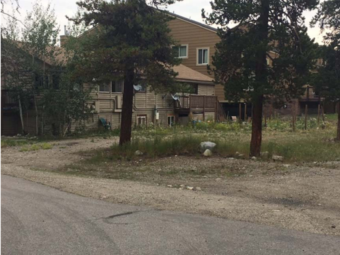
View from southwest corner (August 7, 2017)
