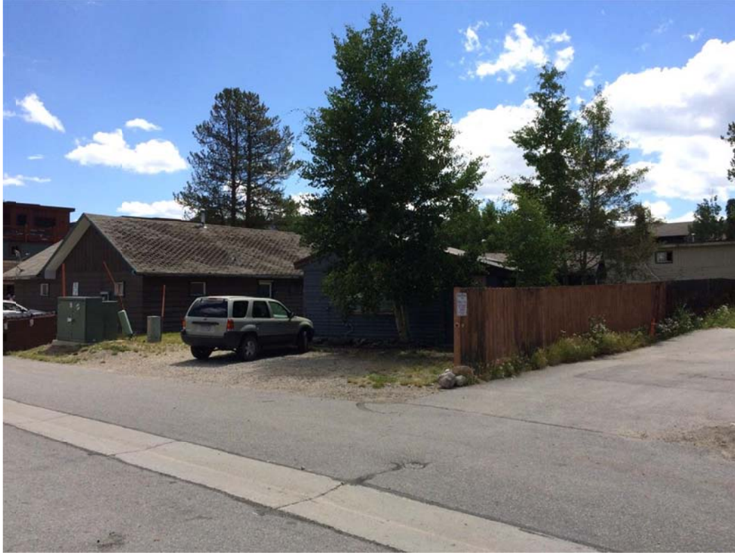
Northwest elevation viewed from Granite Street Alley (8/13/15)
