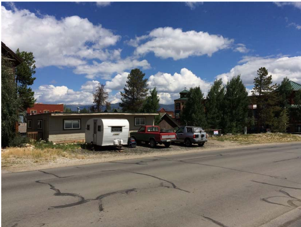
Southwest elevation viewed from Granite Street (8/13/15)
