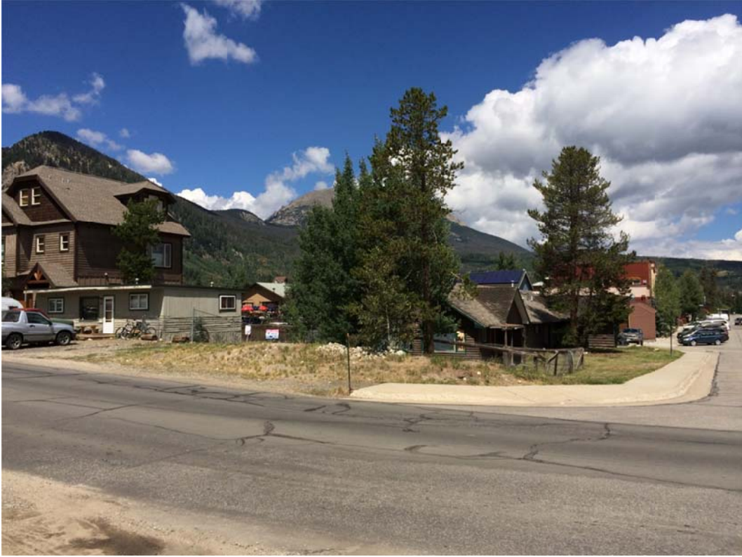
Southeast elevation viewed from Granite Street (8/13/15)
