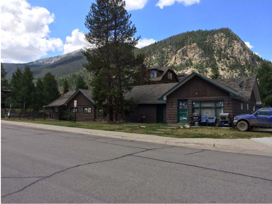
East elevation viewed from South 4 th Avenue (8/13/15)
