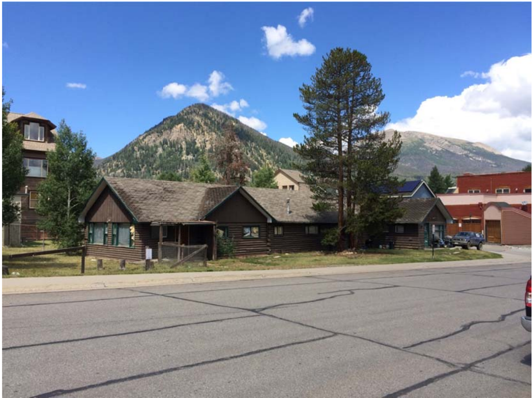
Southeast elevation viewed from South 4 th Avenue (8/13/15)
