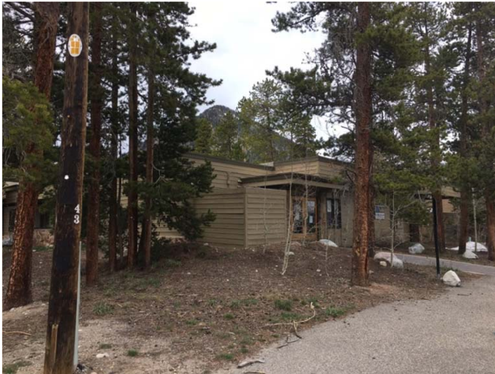
View from southeast corner (04/20/2017)
