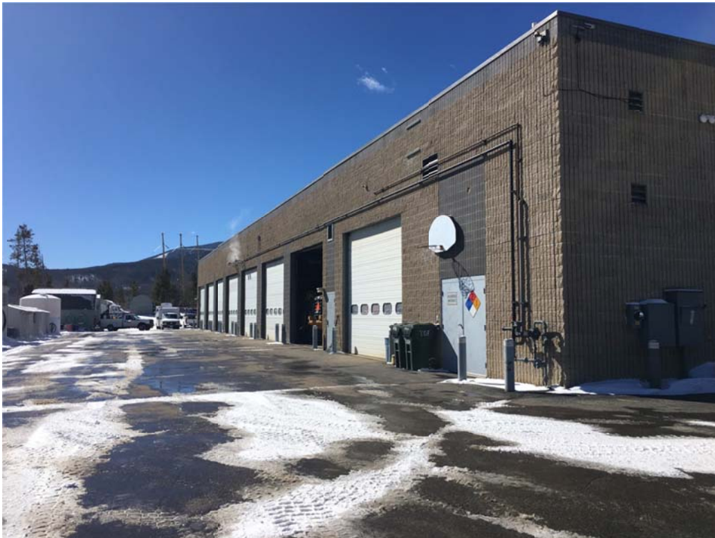
East Façade of Existing Structure
