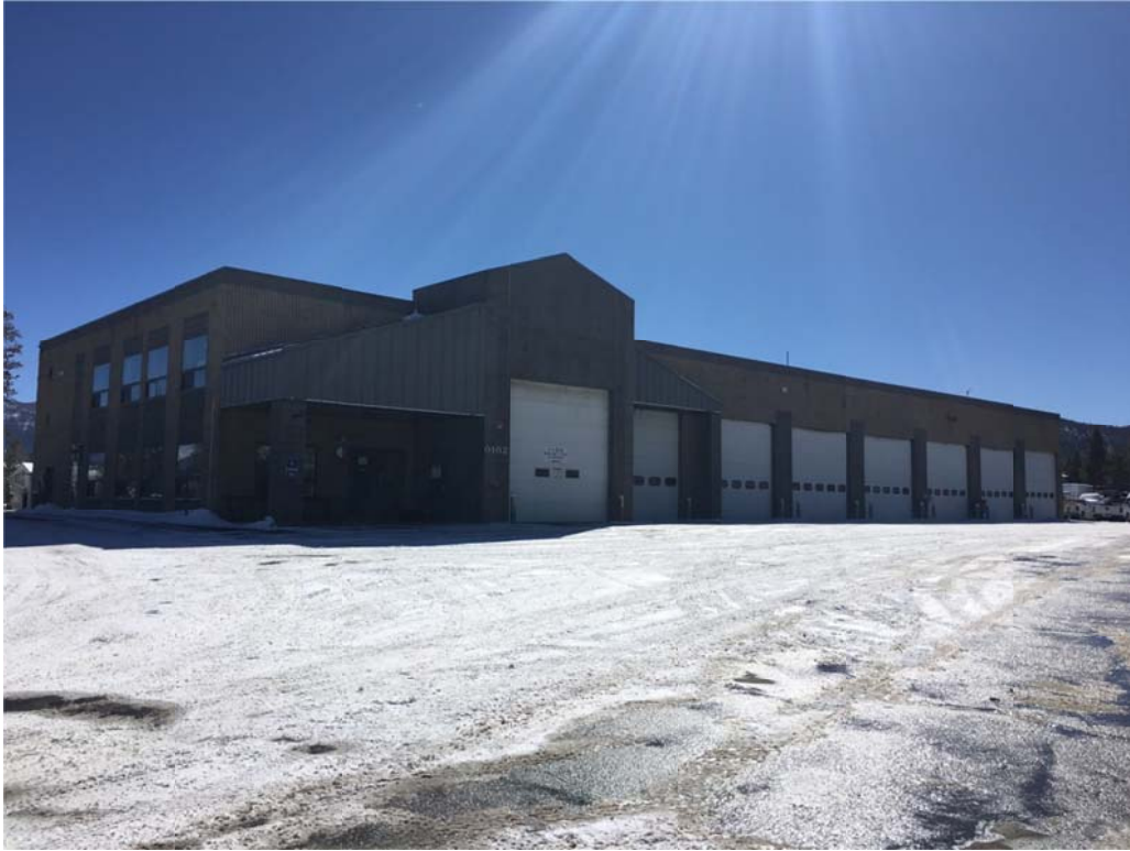
Northwest Corner of Existing Structure
