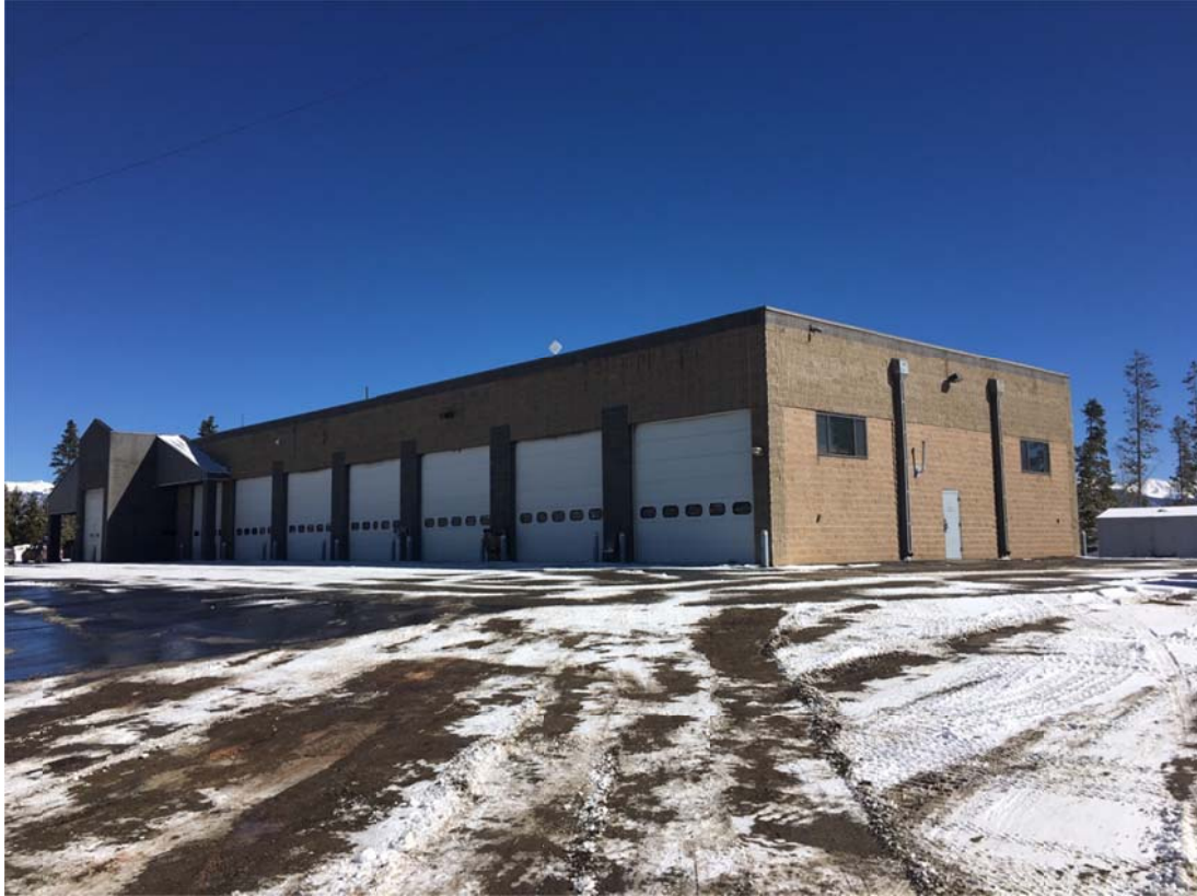
Southwest Corner of Existing Structure
