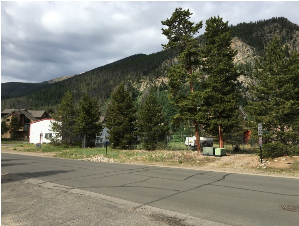
Northeast side from South 2 nd Avenue
