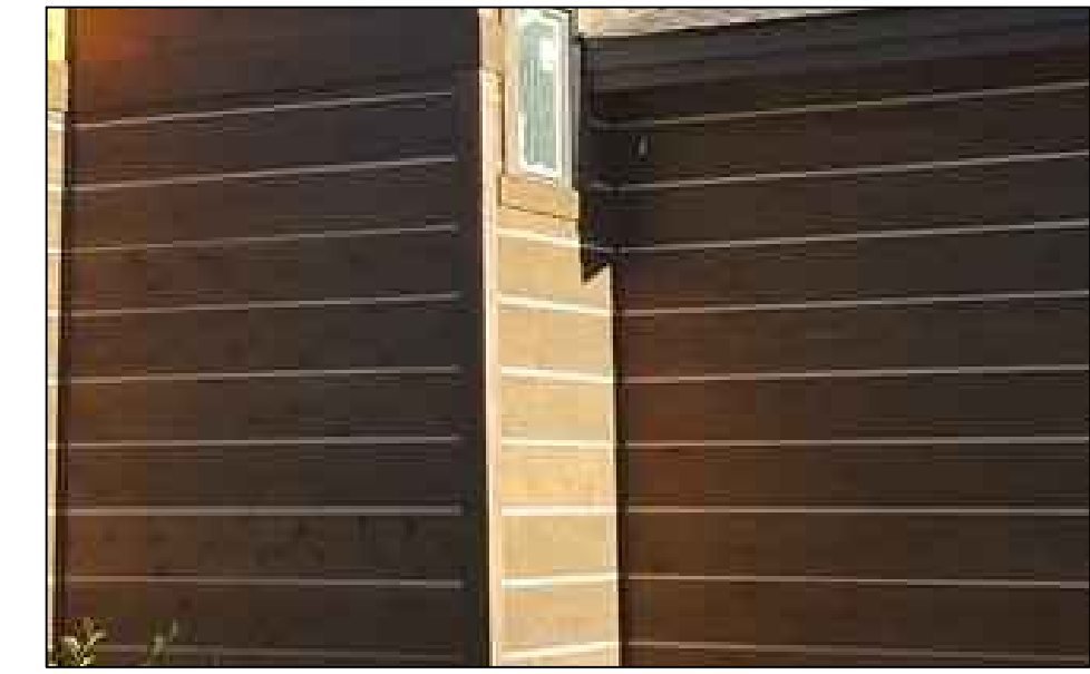
WOOD SIDING FOR UNIT 2 LOWER FLOOR:
