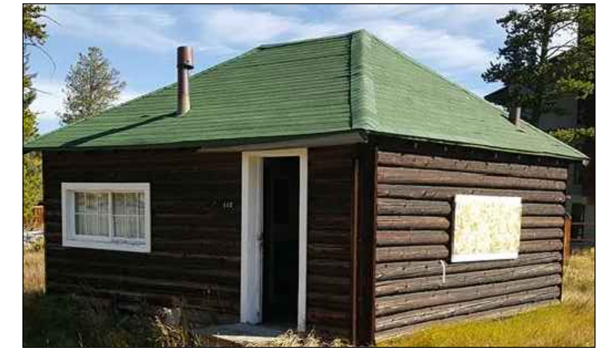
EXISTING DEMING CABIN:
