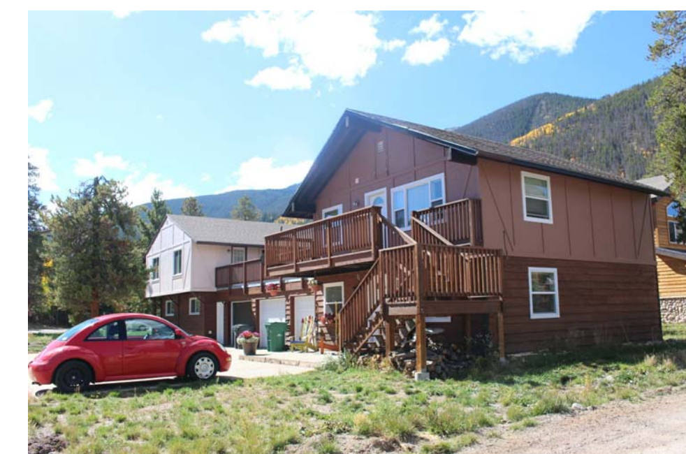
EXISTING DUPLEX AND RESIDENCE, VIEW FROM NORTH-EAST
