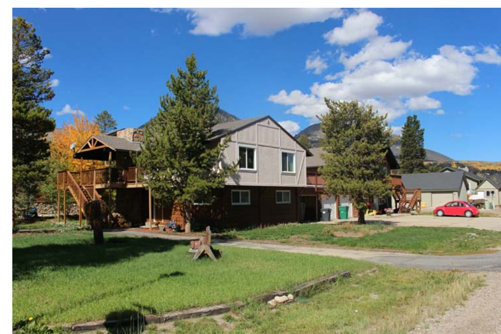
EXISTING RESIDENCE AND DUPLEX, VIEW FROM SOUTH-EAST
