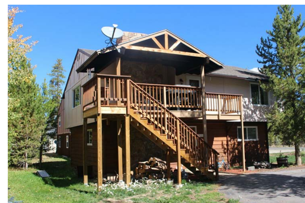
EXISTING RESIDENCE, VIEW FROM SOUTH
