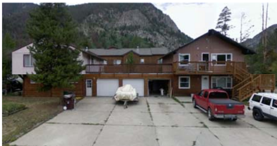
Existing east façade
