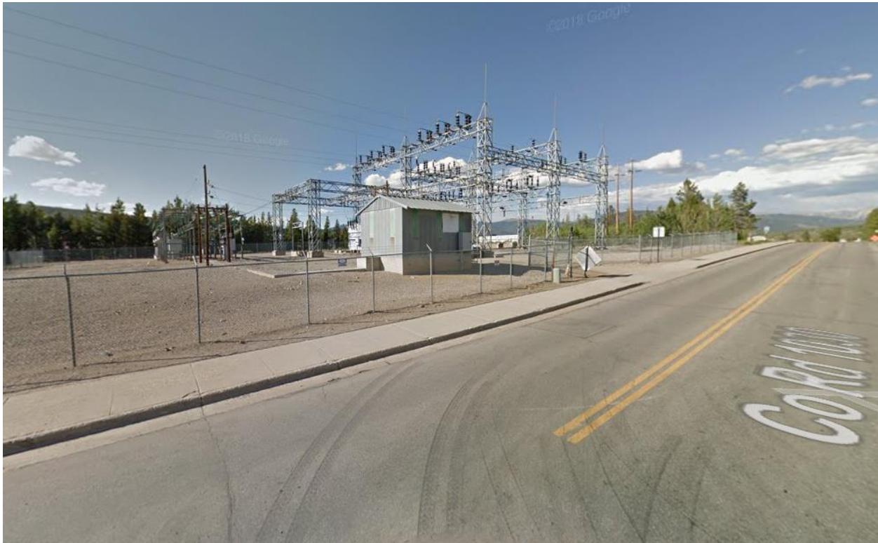
Figure 2. View of Summit Substation, Looking to the northeast
