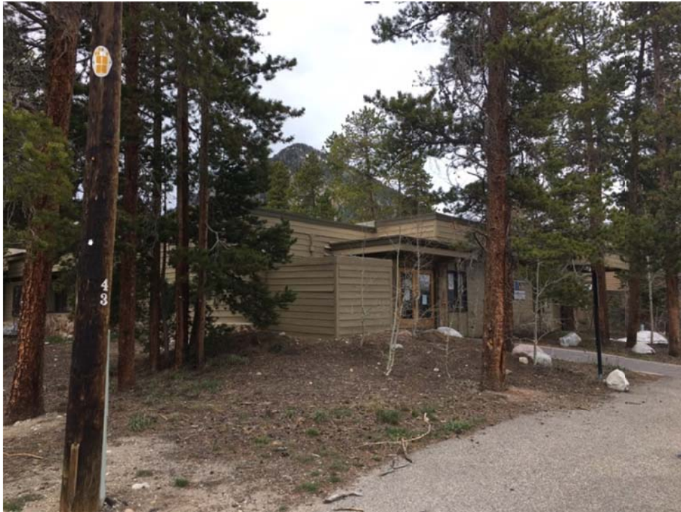
View from southeast corner (04/20/2017)
