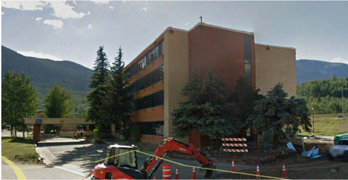
Existing East Façade (Google Earth July 2018)
