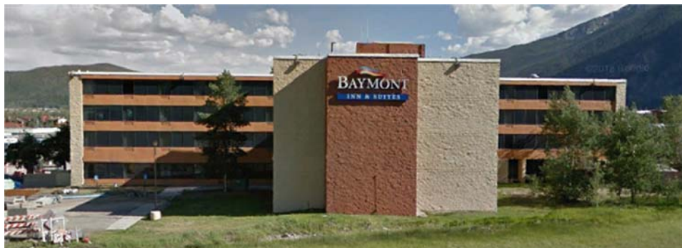
Existing North Façade (Google Earth July 2018)
