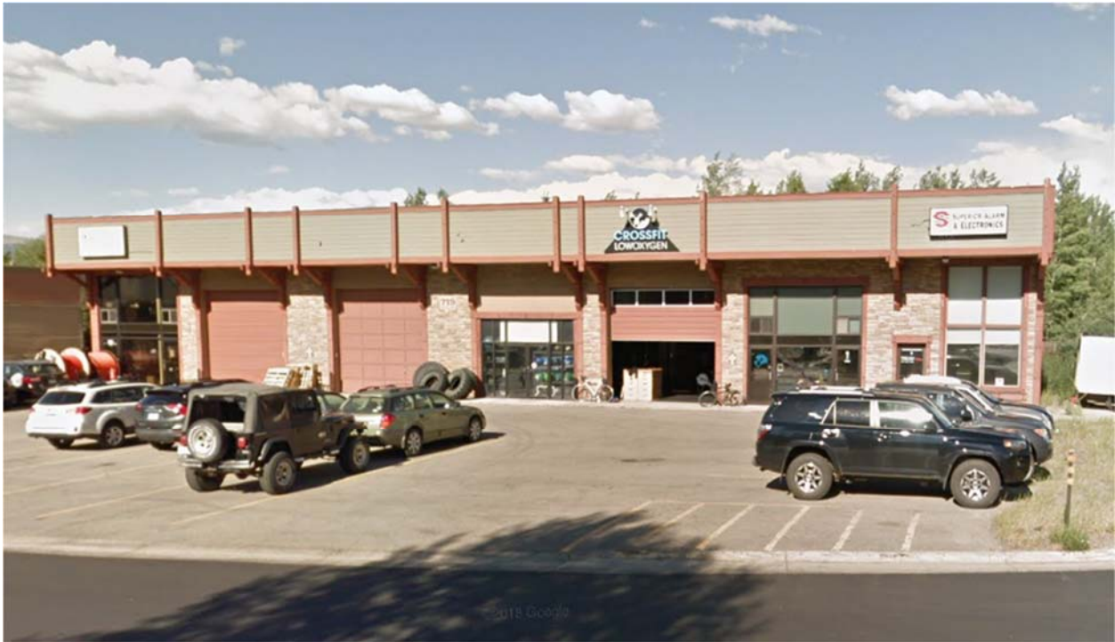
View looking east (Google Earth)
