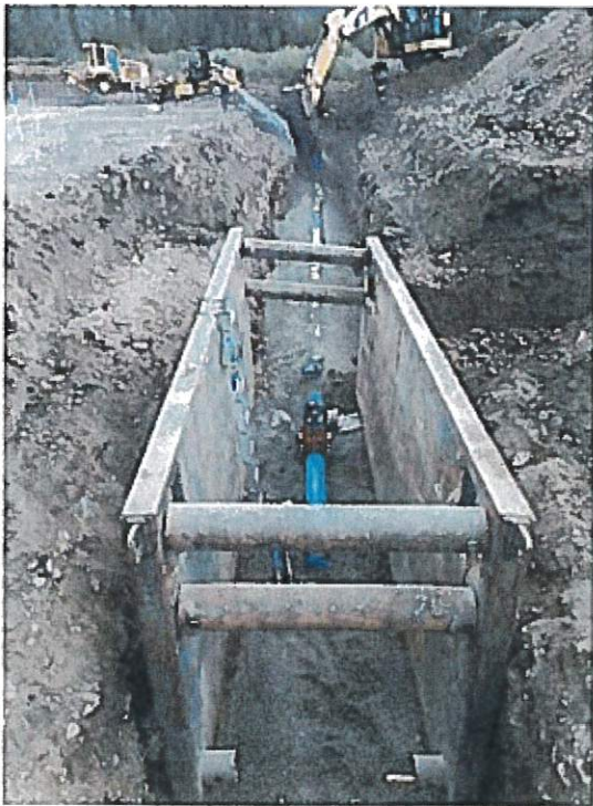
New water main install, Silverthorne, CO
