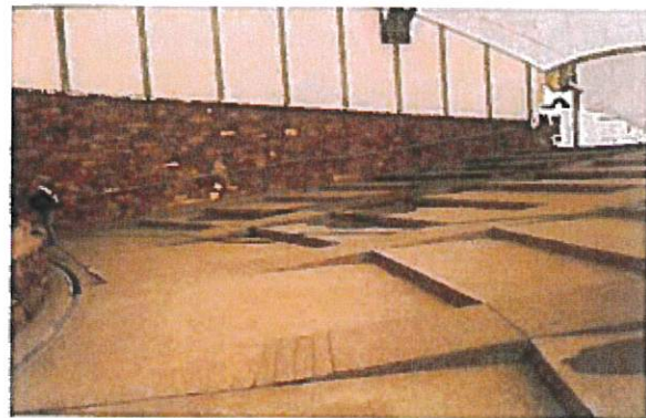
Sloped concrete ramps and stairs at Breckenridge Riverwalk Center.
