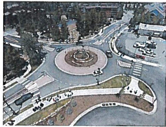
New Round-a-bout constructed for the Town of Breckenridge.
