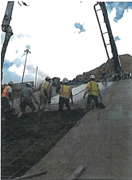
Pouring concrete slope paving on I-70 near the tunnel.
