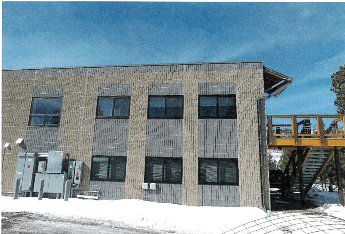
MWGC worked on the Frisco Public Works Office Expansion & Employee Housing Units project in 2018.
