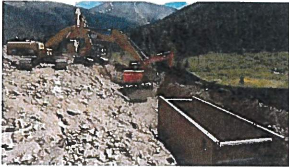
Installation of new reinforced concrete storm pipe and inlets off I-70 near the tunnel.
