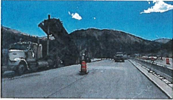
Asphalt Paving for CDOT near Eisenhower Tunnel.
