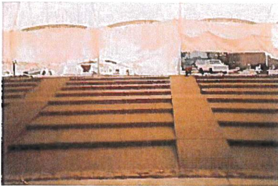
Sloped concrete ramps and stairs at Breckenridge Riverwalk Center.
