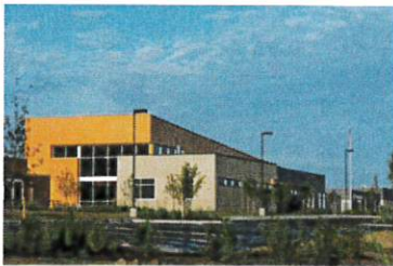
Adams 12 Five Star Schools Transportation Maintenance Facility Thornton
