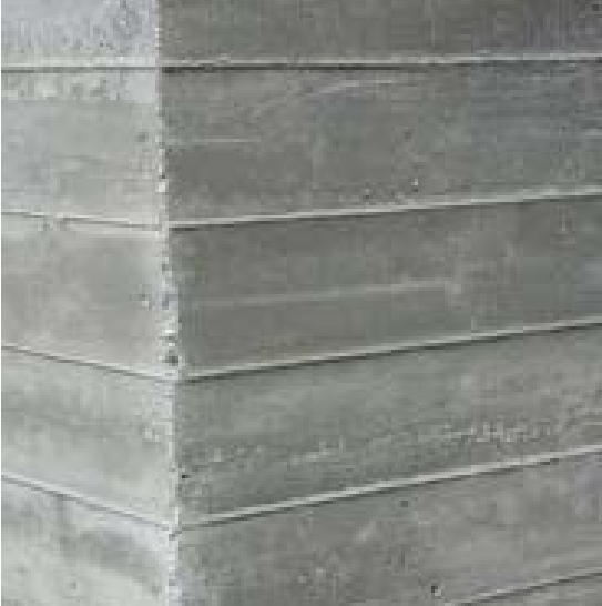
Board Form Concrete
