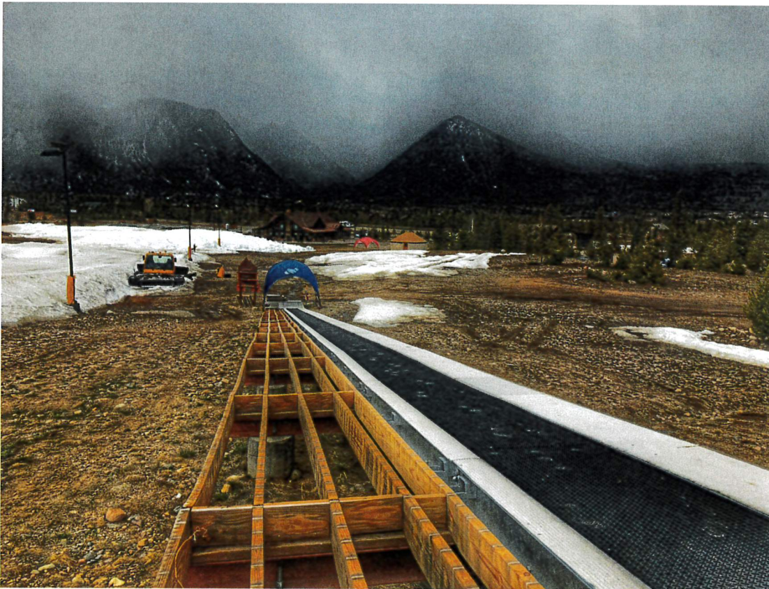
Site from mid-point looking down lift, all wood is being removed by Town
