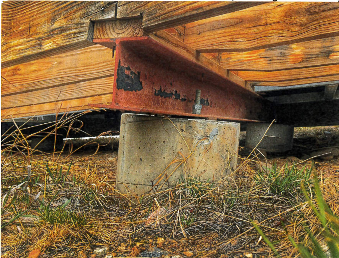
Existing I beam and concrete to be reused, all wood is being removed by Town
