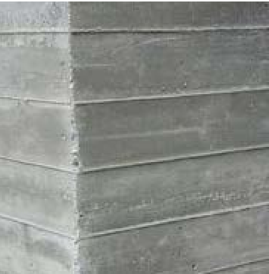
Board Form Concrete
