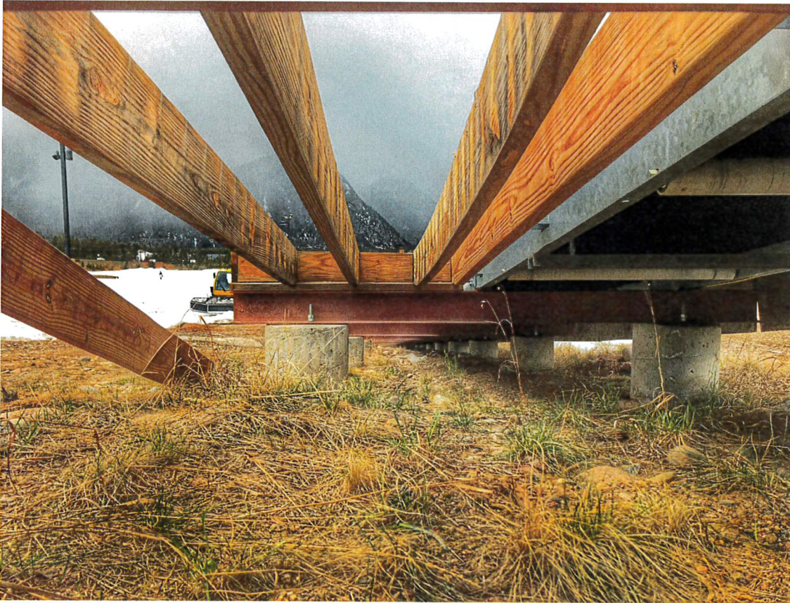
Another view of I beam on concrete supports
