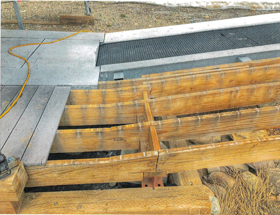
Transition to lower deck, wood to the left to remain, to the right removed by Town
