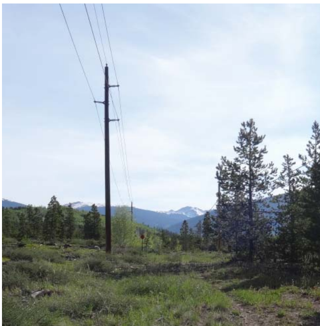
Site photo, view northeast
