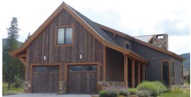
Wood siding / typical Frisco roof form
