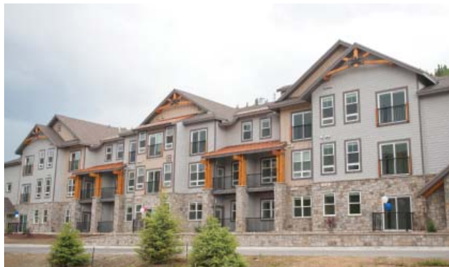
Timber columns and brackets
