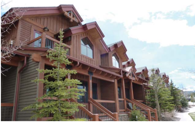
Brackets and heavy timber columns at porch / patios
