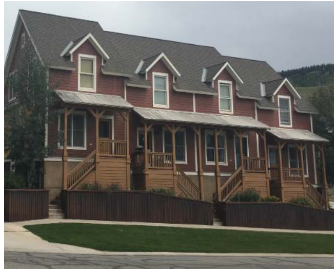
Front porches on townhomes, Pitchfork Affordable Housing, Crested Butte, CO
