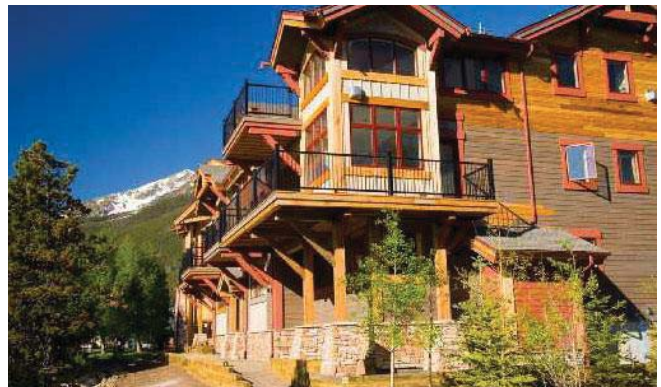
Varying roof form / substantial trim elements / timber columns and brackets
