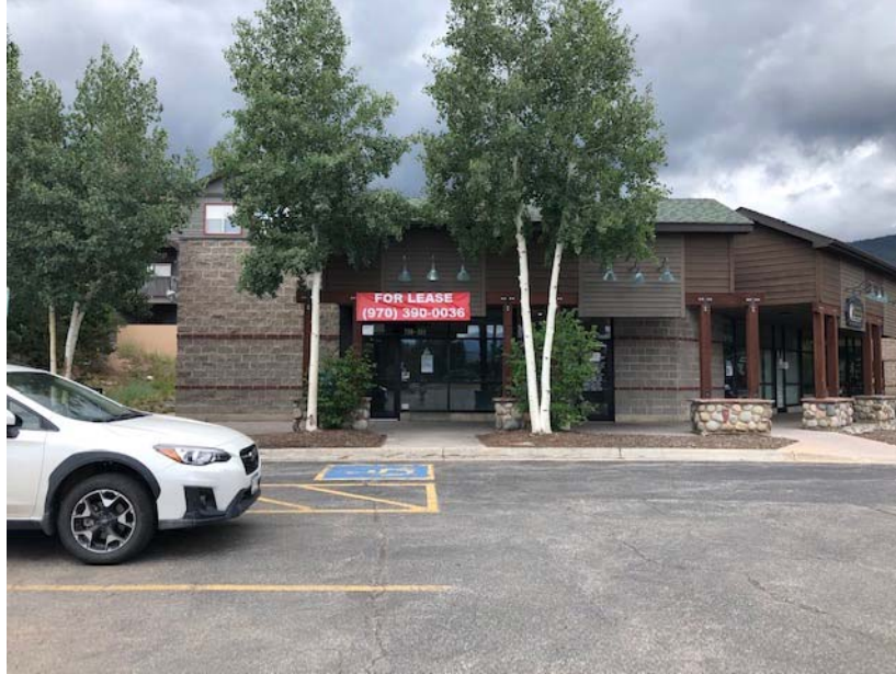
View looking west at unit (July 28, 2020)
