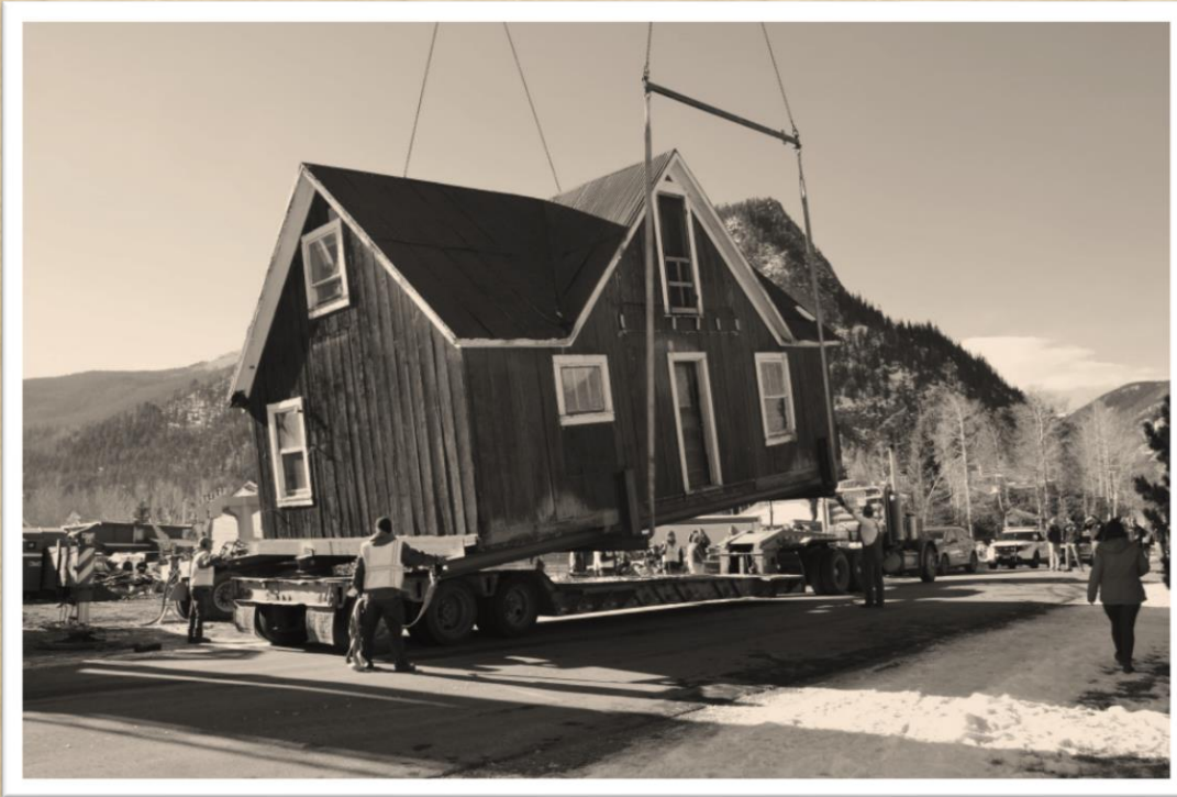
Excelsior Mine Office Building Preservation Project 2018
