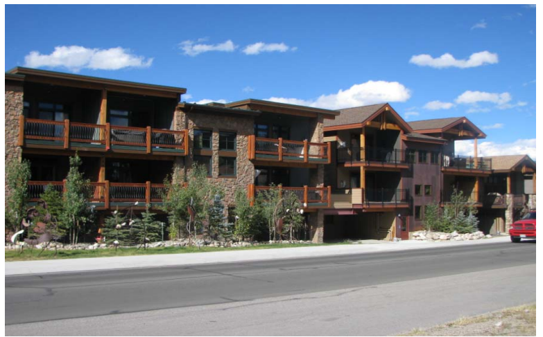
Southern elevation of building and view of site looking northeast over Granite Street from Corner of 4th and Granite St.
