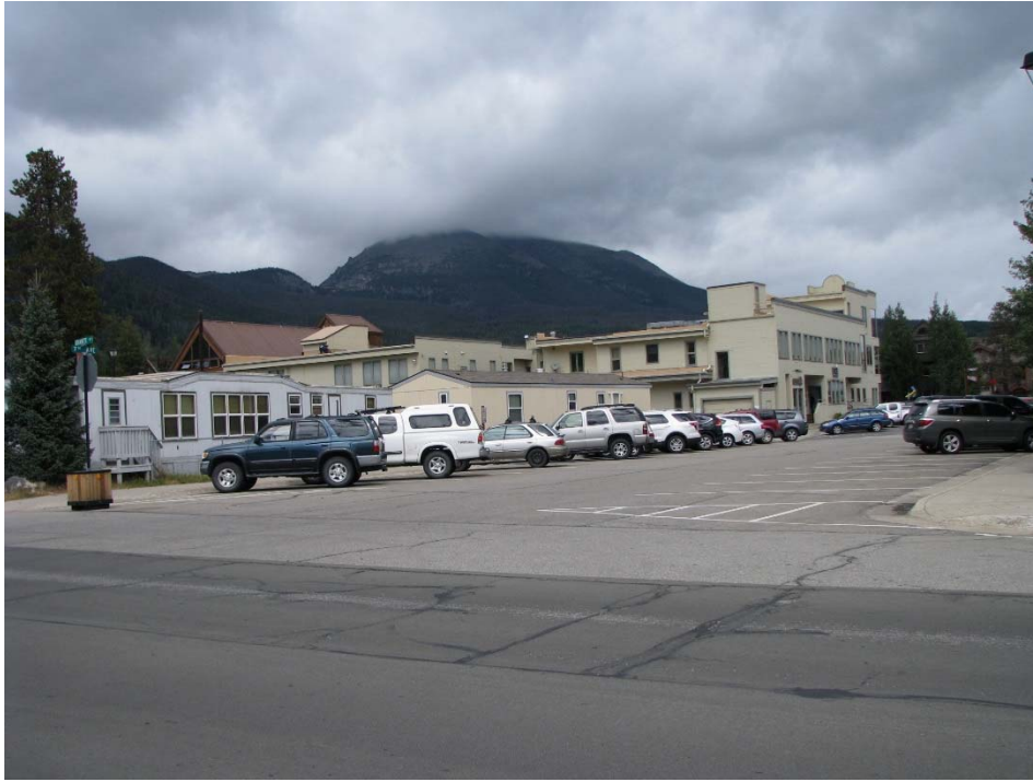
Southeastern corner of subject looking northwest from the intersection of S. 7 th Avenue and Granite Street
