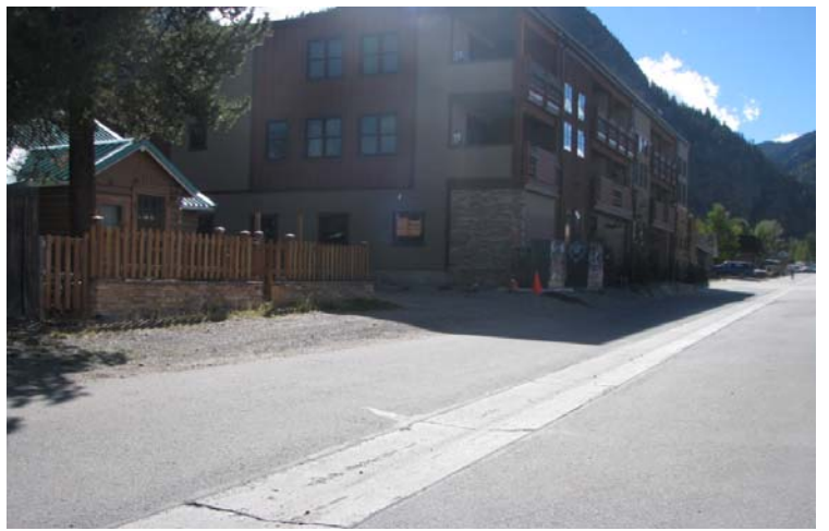
Alley view looking west at northern elevation of building
