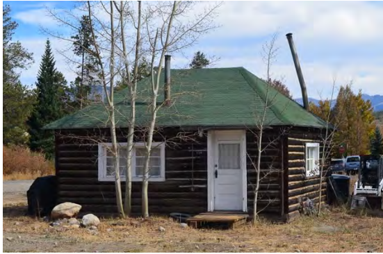
116 N 5th Ave • 5ST.1746 • Deming Cabin 1938 • This cabin is associated the Deming family, who were an important members of early Frisco society. The construction of the cabin includes an inverted corner detail, which seems to be a common detail in Frisco.
