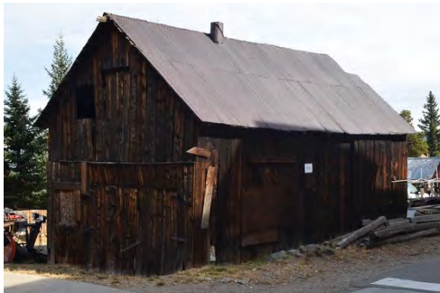
502 Main St • 5ST.1764 • Blacksmith 1920s • This building appears to be in original condition with some of the smithing adaptations still intact. It is part of an approved development plan that will preserve some of the character of this building.
