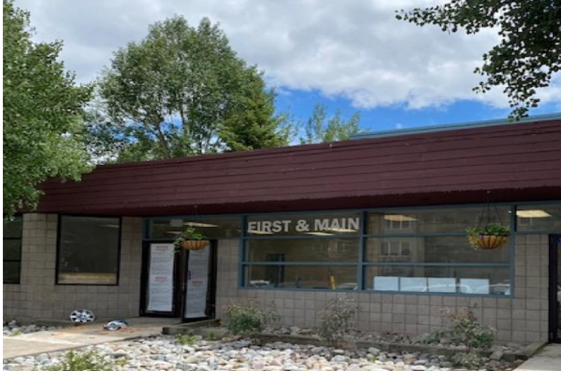
1 st and Main Building
