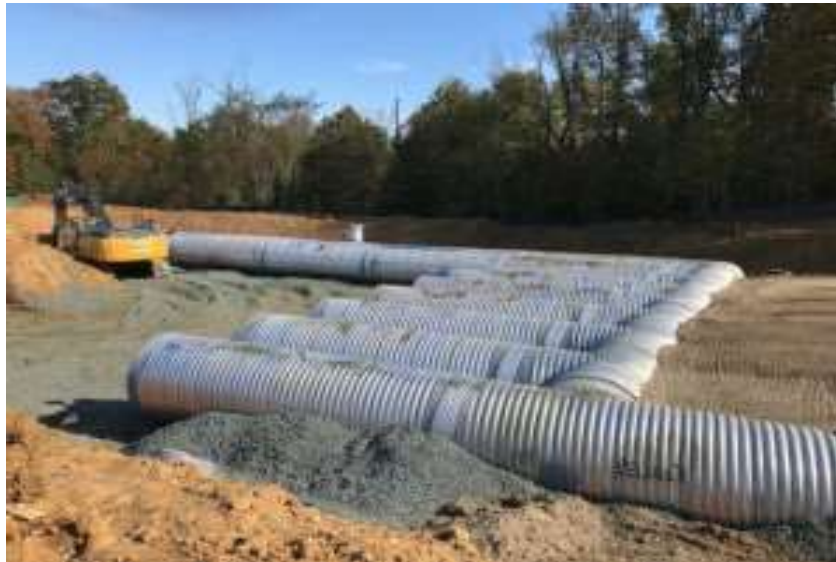
Storm Water Pipes
