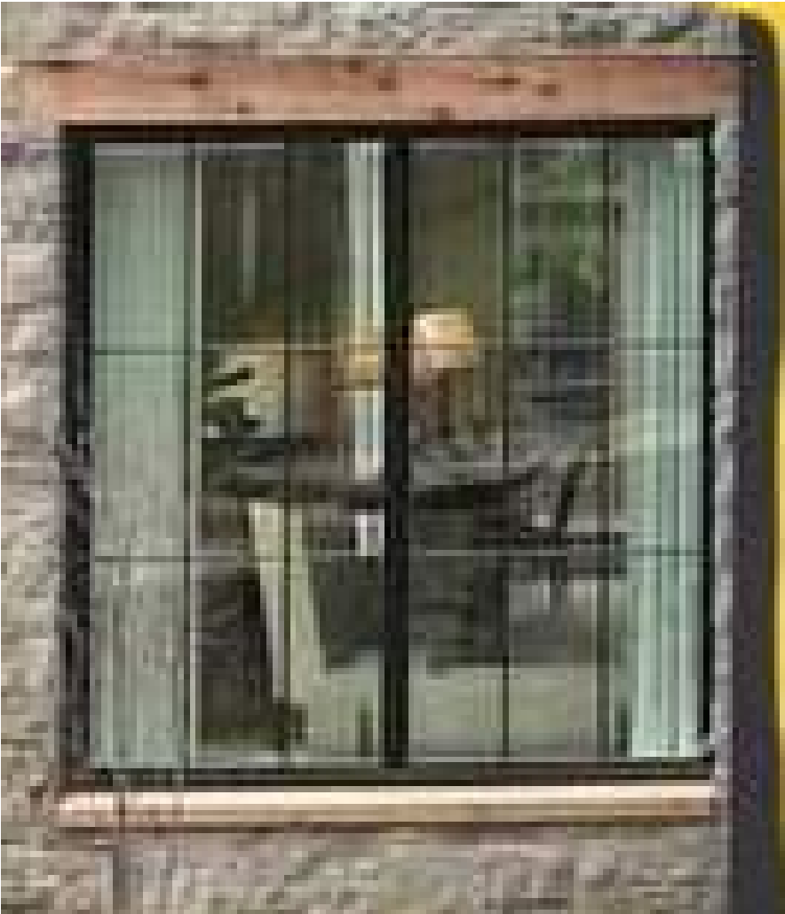
14. 10" TIMBER HEADER IN STONE VENEER
