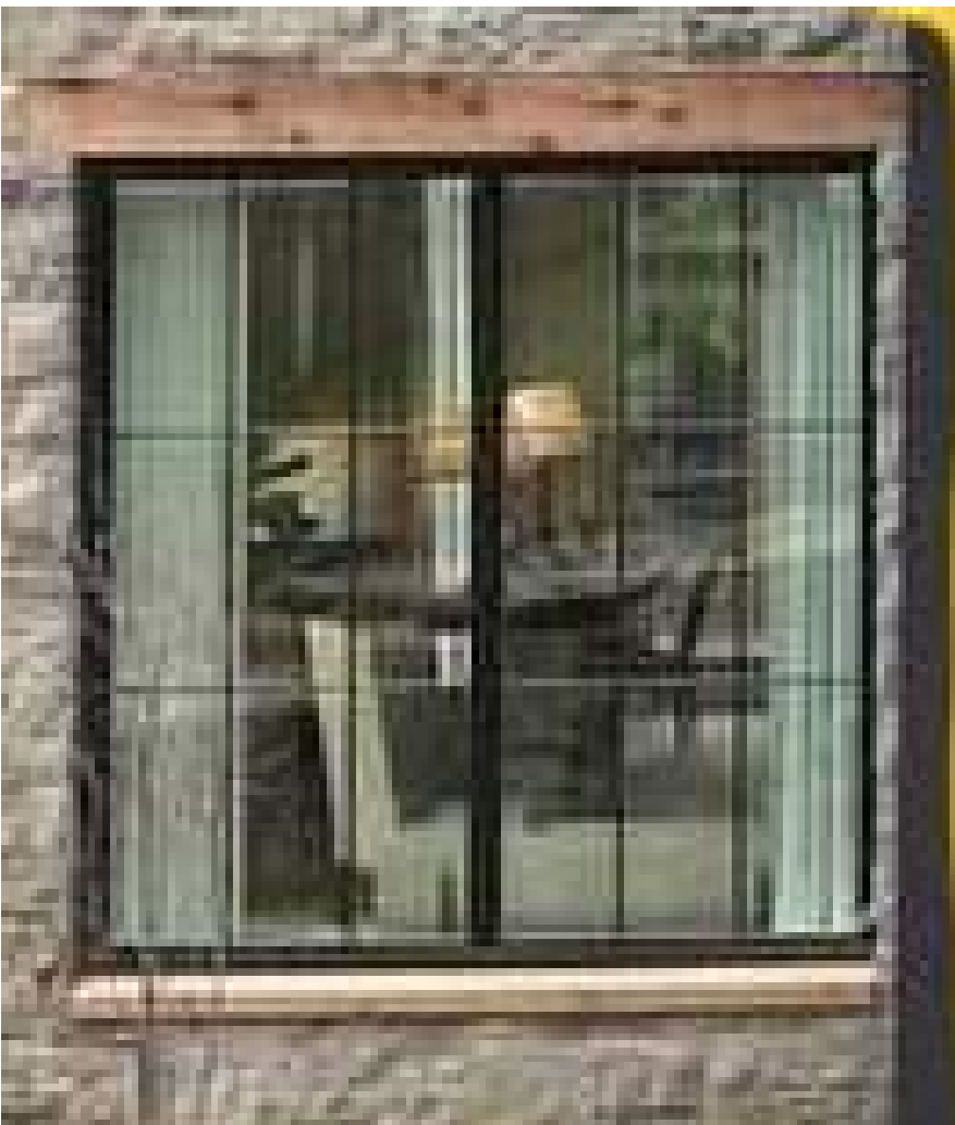
14. 10" TIMBER HEADER IN STONE VENEER
