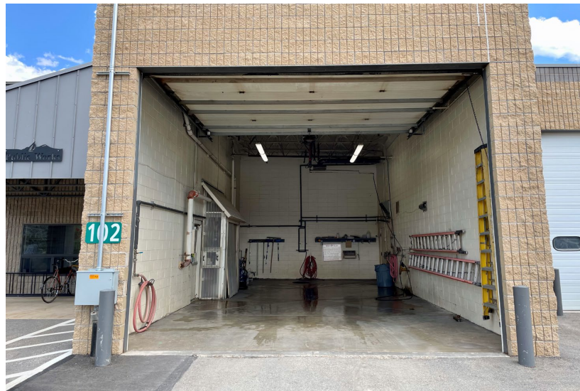
Public Works Wash Bay
