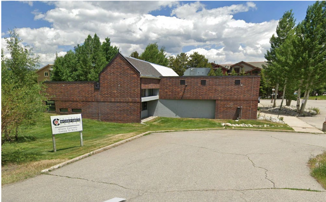
Existing Condition of Facility from 6th Ave.
