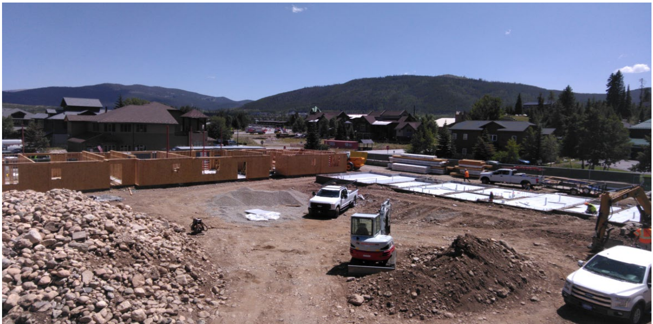
Framing on East Building and Foundation on West Building
