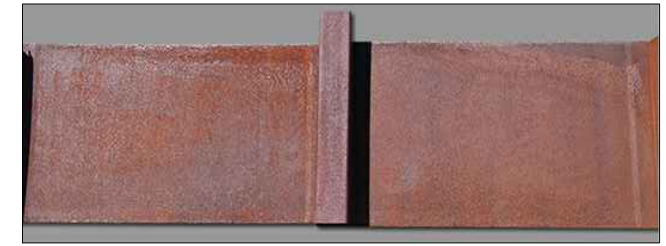
STANDING SEAM METAL ROOF
